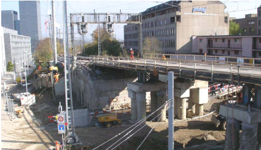
■ Reconstruction of the 100 years old railway bridge carrying two railtracks.
