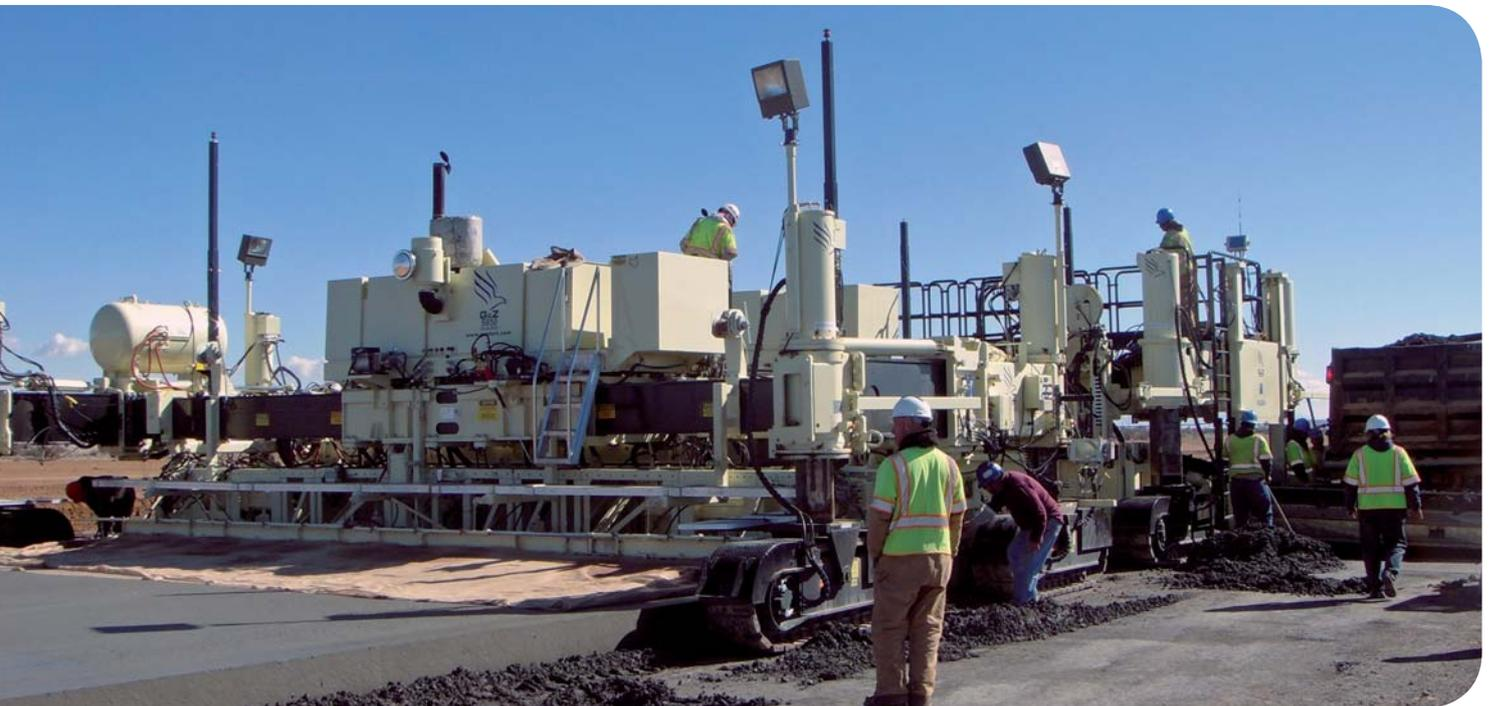
■ Montoya is paving the runway with a Guntert & Zimmerman S850 slipform concrete paver automatically controlled by a Leica PaveSmart 3D system.
